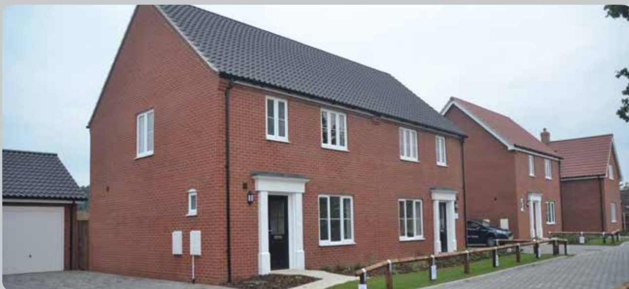
One of the houses at the Rosebery Park development, which is being built by Big Sky Developments – a company wholly-owned by South Norfolk Council. The final development will consist of 57 two, three and four bed houses.
