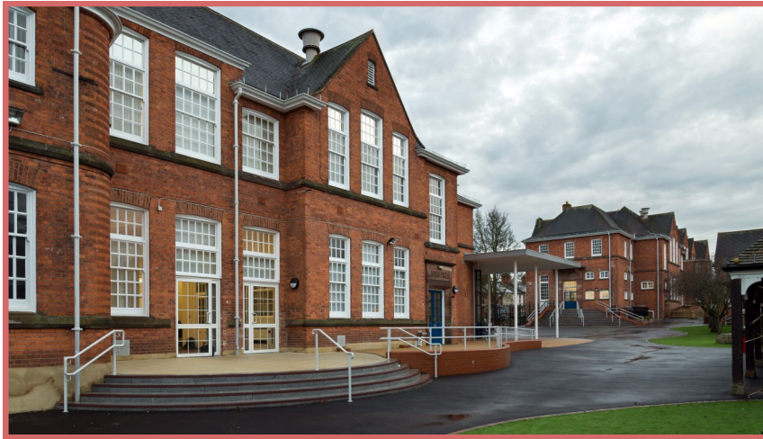
Wilson Primary School, Reading Borough Council
